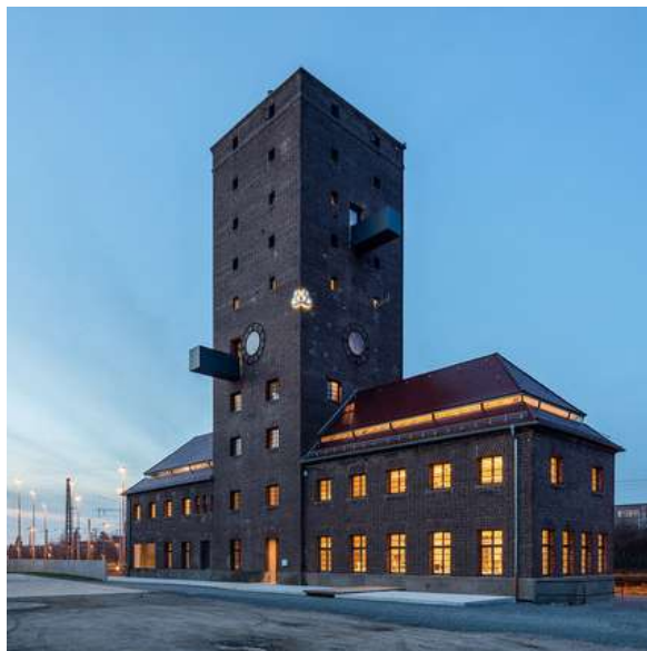
Tankturm, Heidelberg © Thomas Ott
