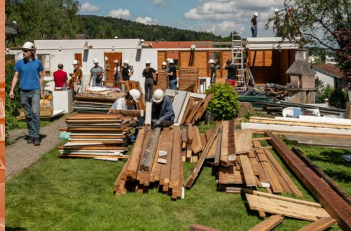
Disassembly of Oetwil am See Music Pavillion for Reuse © Buser Hill Photography, CEA lab
